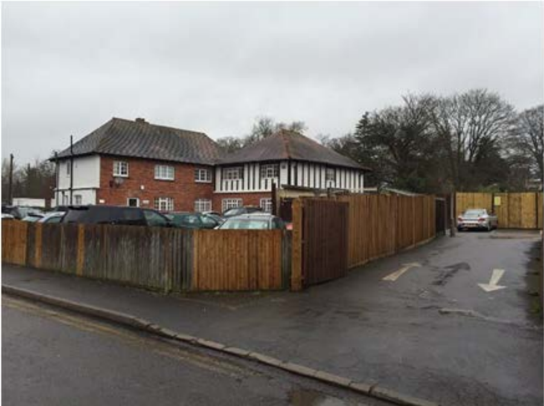
River Walk Offices looking north west
